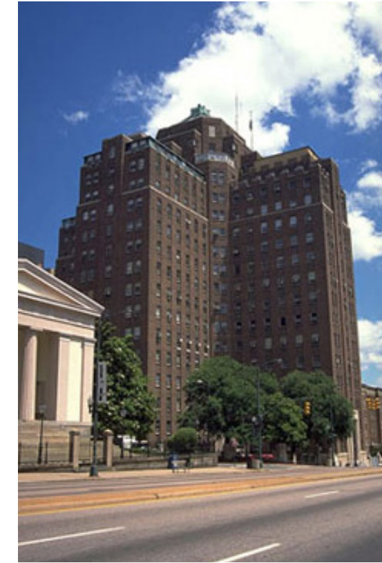
exterior view from broad street
